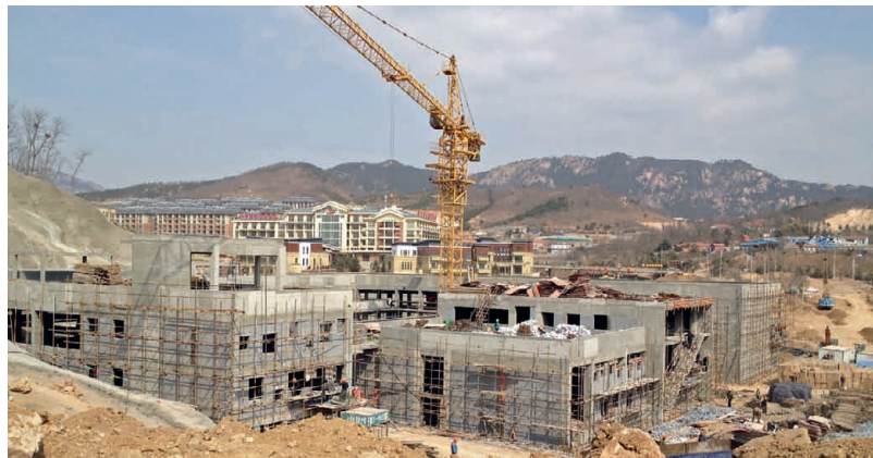
7. STC construction site, Qingdao, March 2014
